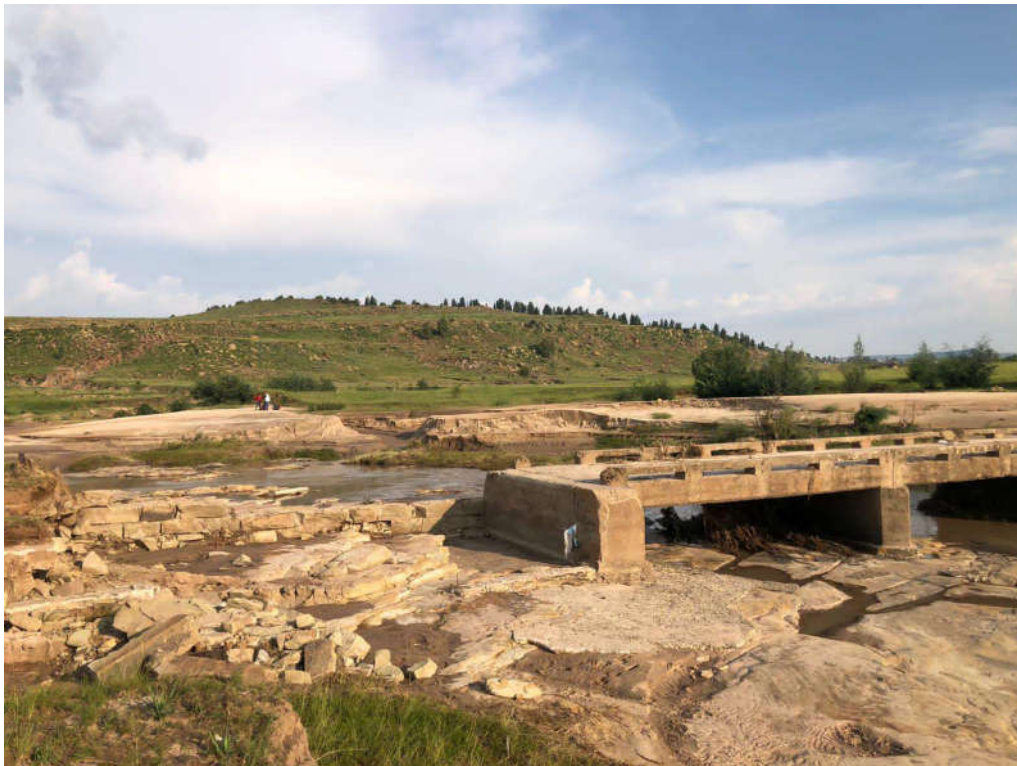
Photo 7: Vented fords crossing 1 undermined by floods
