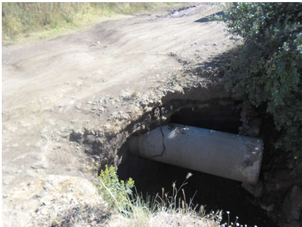
Photo 13: Silted 600 diameter pipe and overtopping plate
