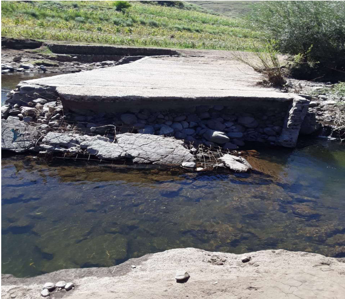
Photo 5: Damaged vented ford crossing filled with rocks and lined with concrete reinforced with mesh as a slab with stone masonry walls
