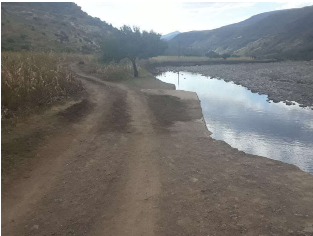
Photo 9: B44 road cut off at Ha Masiu as river meandered Community fields being used as temporary deviation
