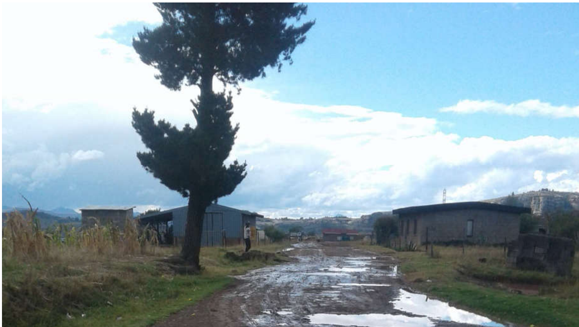
Photo 15: minimal grade resulting in potholing due to insufficient drainage
