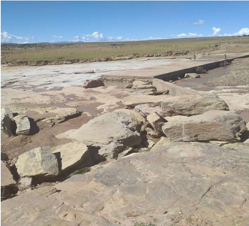
Photo 8: Vented fords crossing 2 undermined by floods
