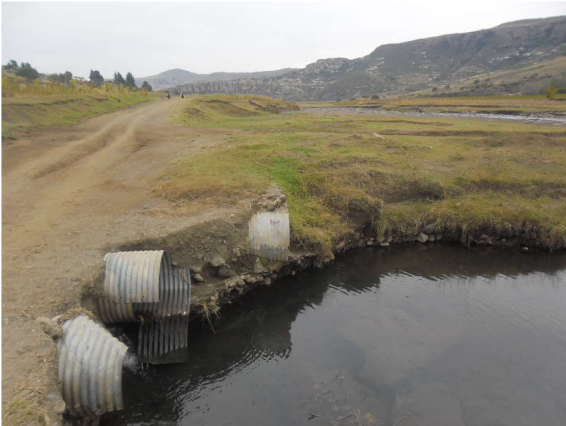
Photo 6: Substandard vented ford crossing with blocked culverts, gravel loss and vented ford not constructed to Roads Directorate Standard
