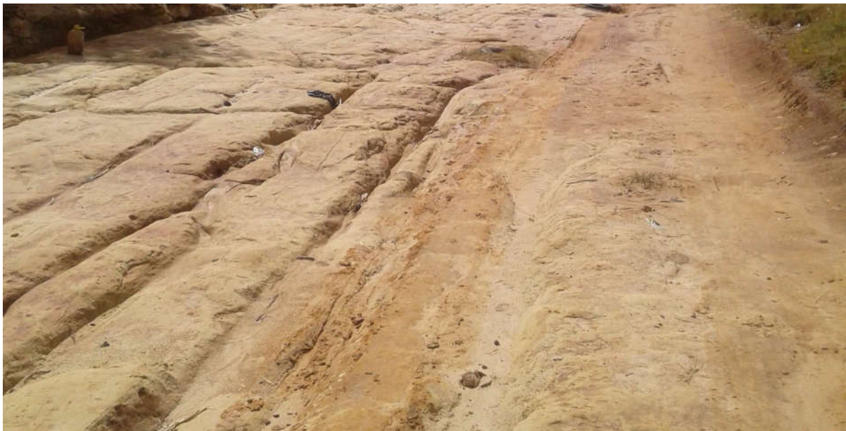
Photo 17: Gravel loss on sandstone outcrop
