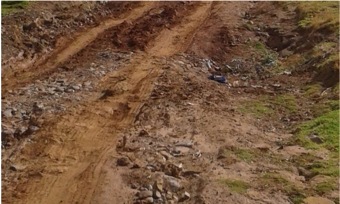
Photo 16: Gravel loss between 1+900 and 5+000
