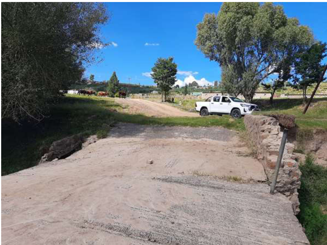
Photo 2: Vented ford structure 1 crossing at Machekoaneng River
