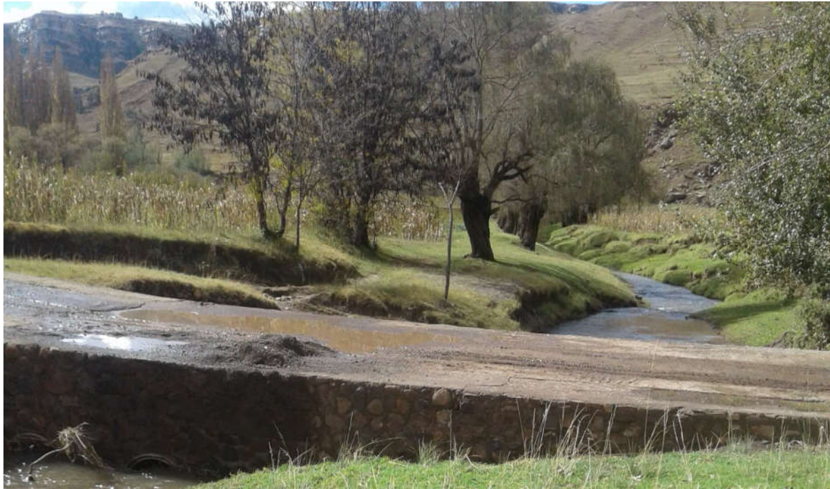
Photo 18: Stream meandering and culverts blocked as a result of meandering
