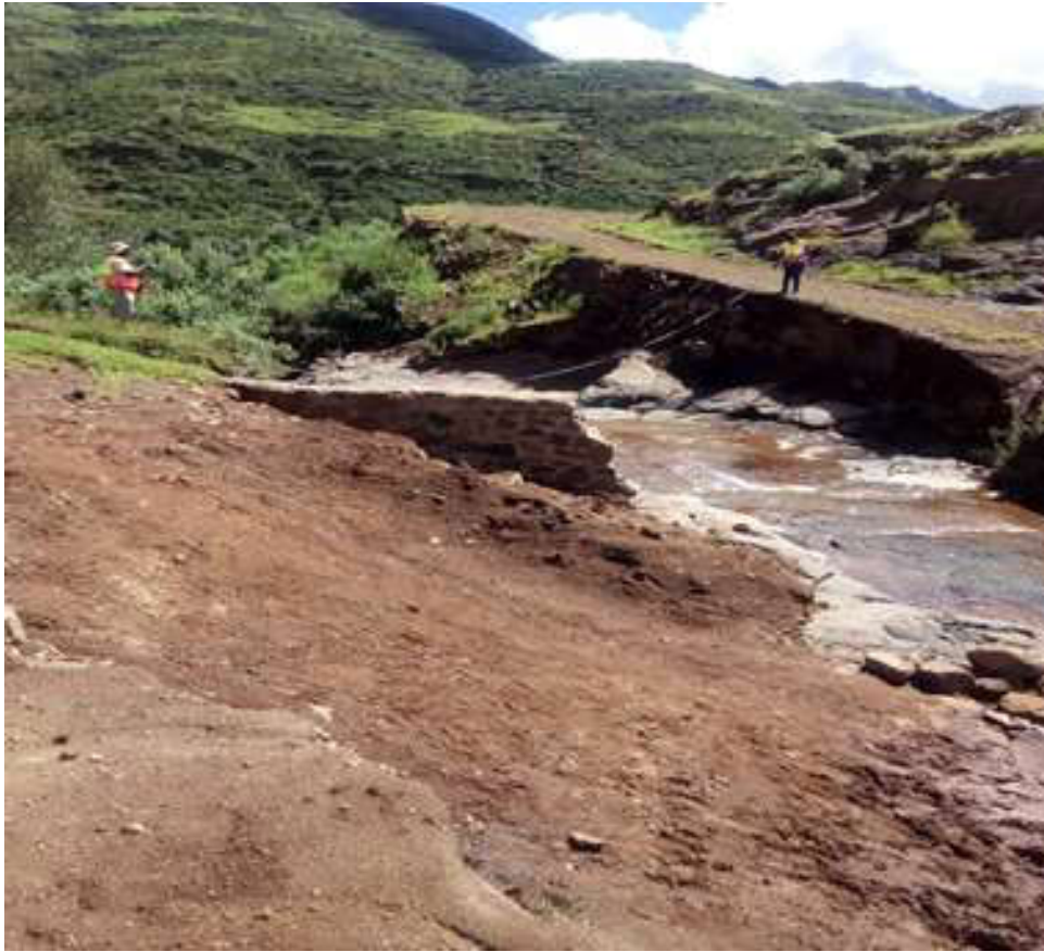
Photo 20: Headwall constructed on solid rock without any rock dowels for anchor
