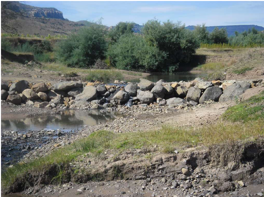
Photo 4: Temporary crossing constructed from Dump Rip Rap
