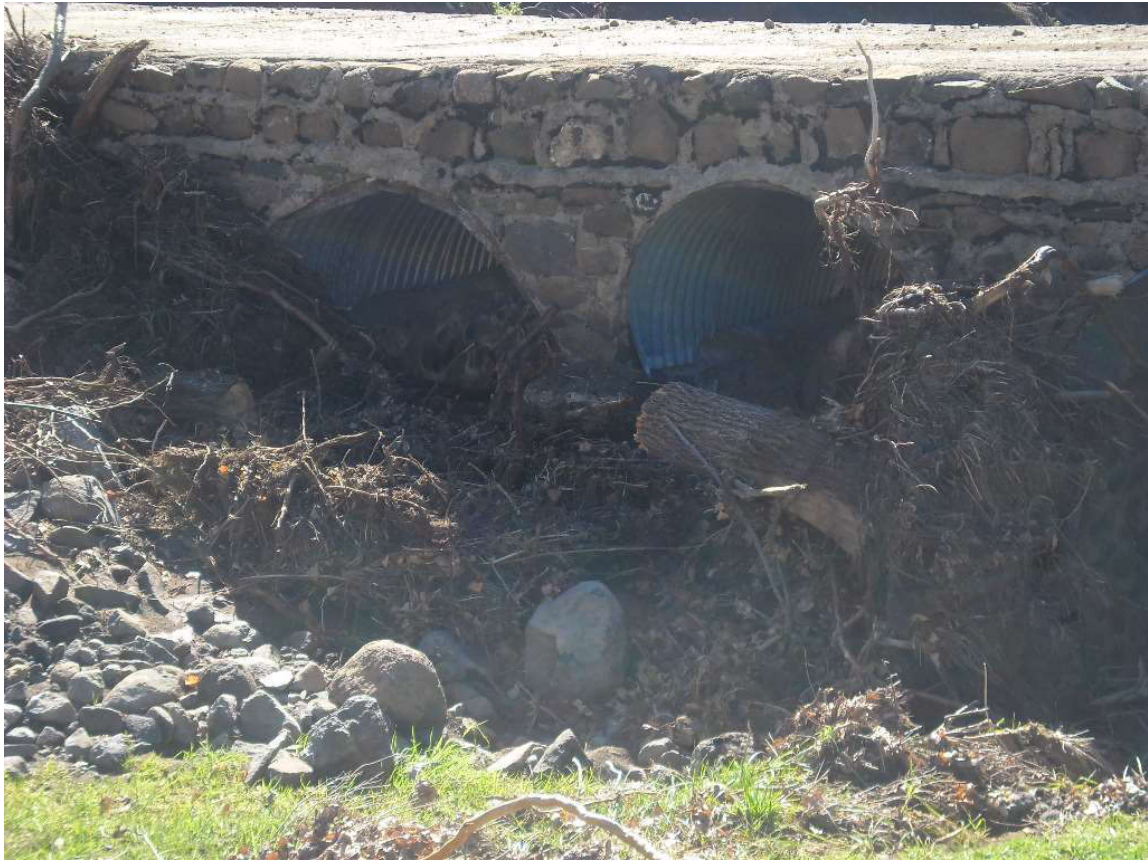
Photo 11: Mini Bridges blockage from debris on upstream side while openings not blocked on the downstream side on Basalt
