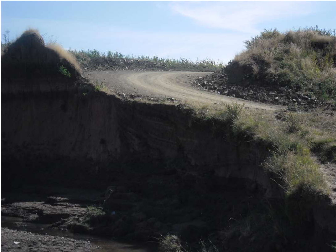
Photo 3: River Bank on meandering section of the River being eroded which will eventually result in road being compromised
